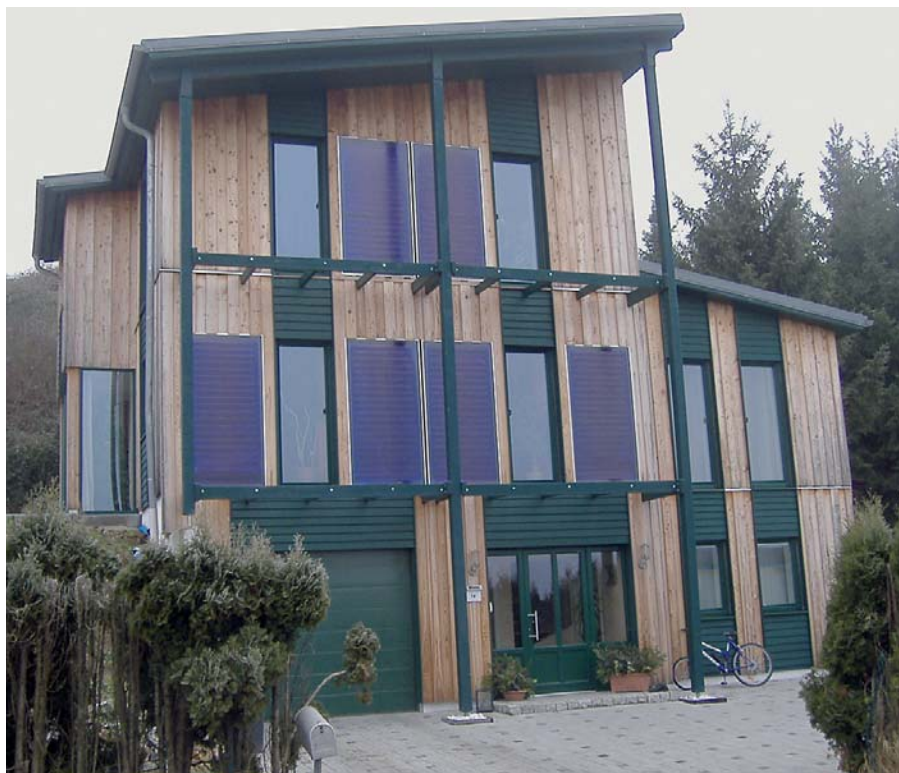
Passivhaus in Mitterfels
